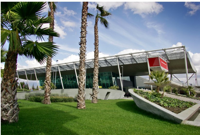
Nene Tereza Airport after reconstruction
